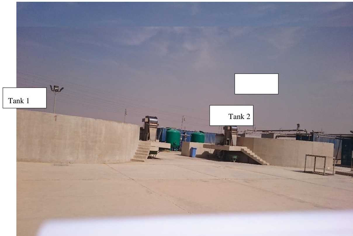
Figure 23: Madinaty- Water Storage Tanks
