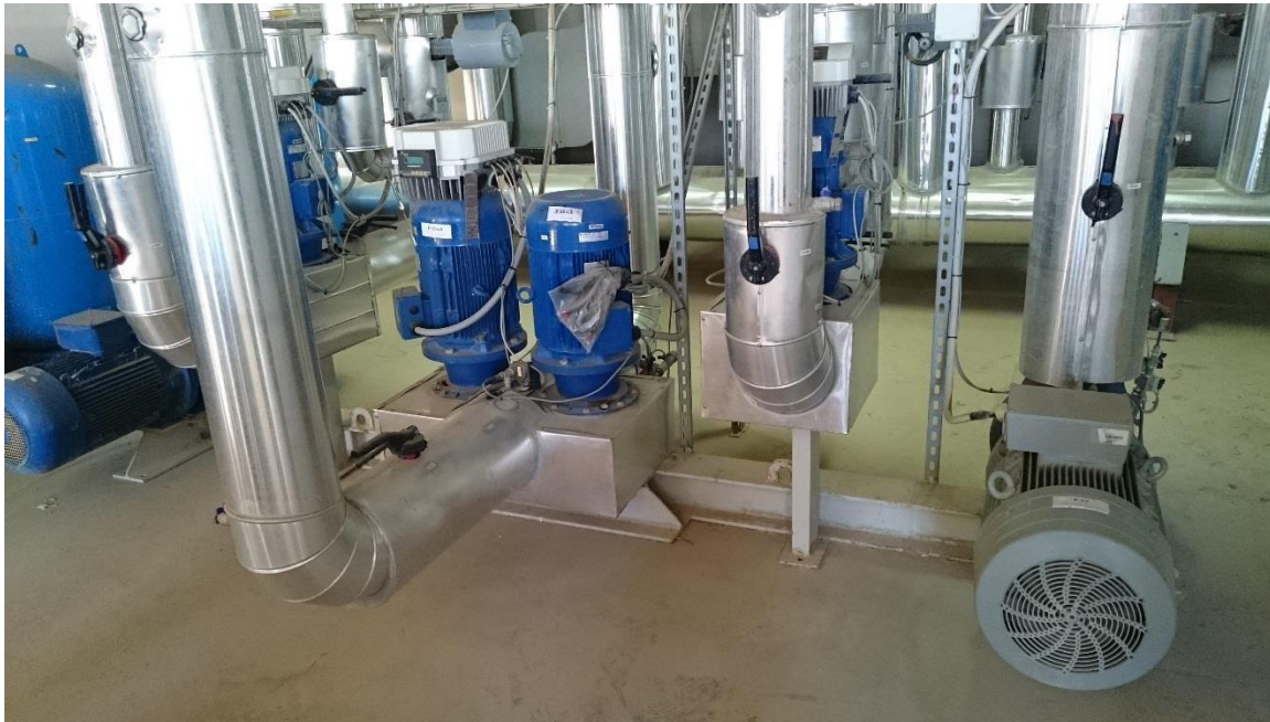
Figure 21: Solar Panels Motors and Pumps
