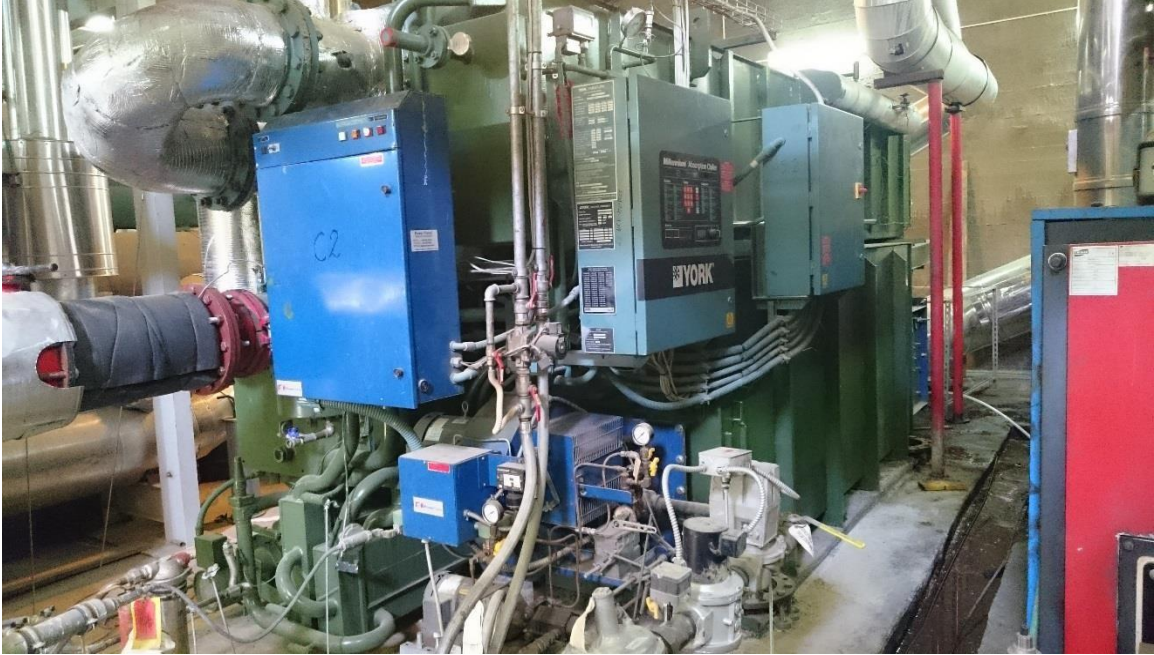
Figure 2: High Capacity Chiller/ Large Tonnage Chiller (LTC)
