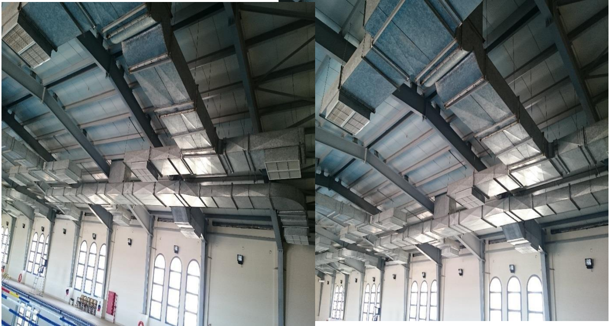
Figure 8: Non- Decorative Ceiling Ducts
